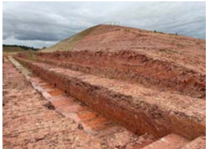
Figure 5 Deconstruction of the trial embankment
