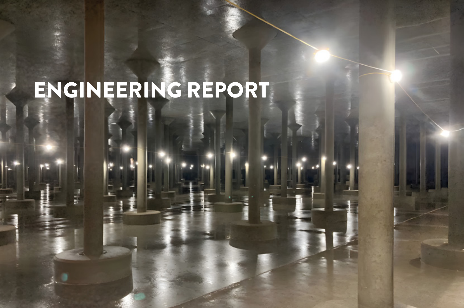
Reservoir inspection and maintenance in progress
