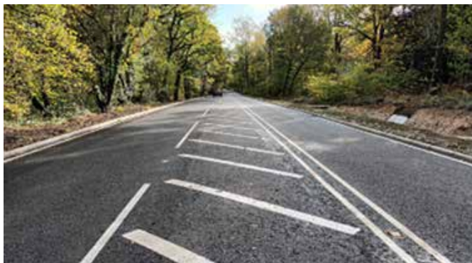
Figure 8 Works to the B2149 has improved safety ahead of creating a new junction for a northern access route to the site
