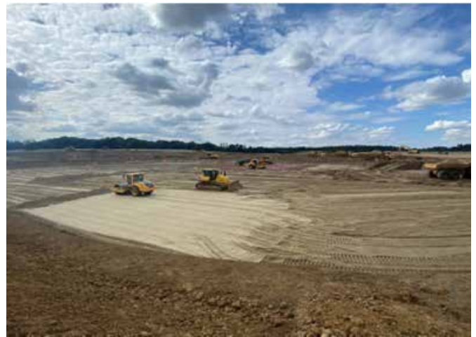
Figure 5 Construction Works on 250mm sand drainage blanket for the Trial Embankment
