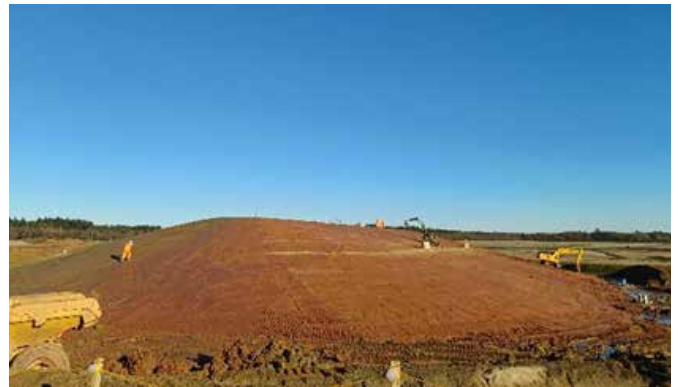
Figure 6 Trian embankment completed on 3 December and subject to ongoing monitoring
