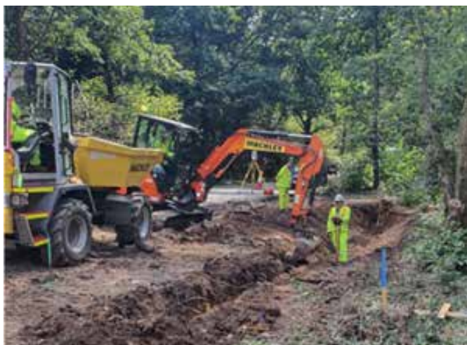
Figure 7 Construction Works on the re-alignment of the B2149 highway
