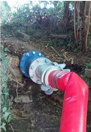
Temporary pipework connection (12/08/2022)
