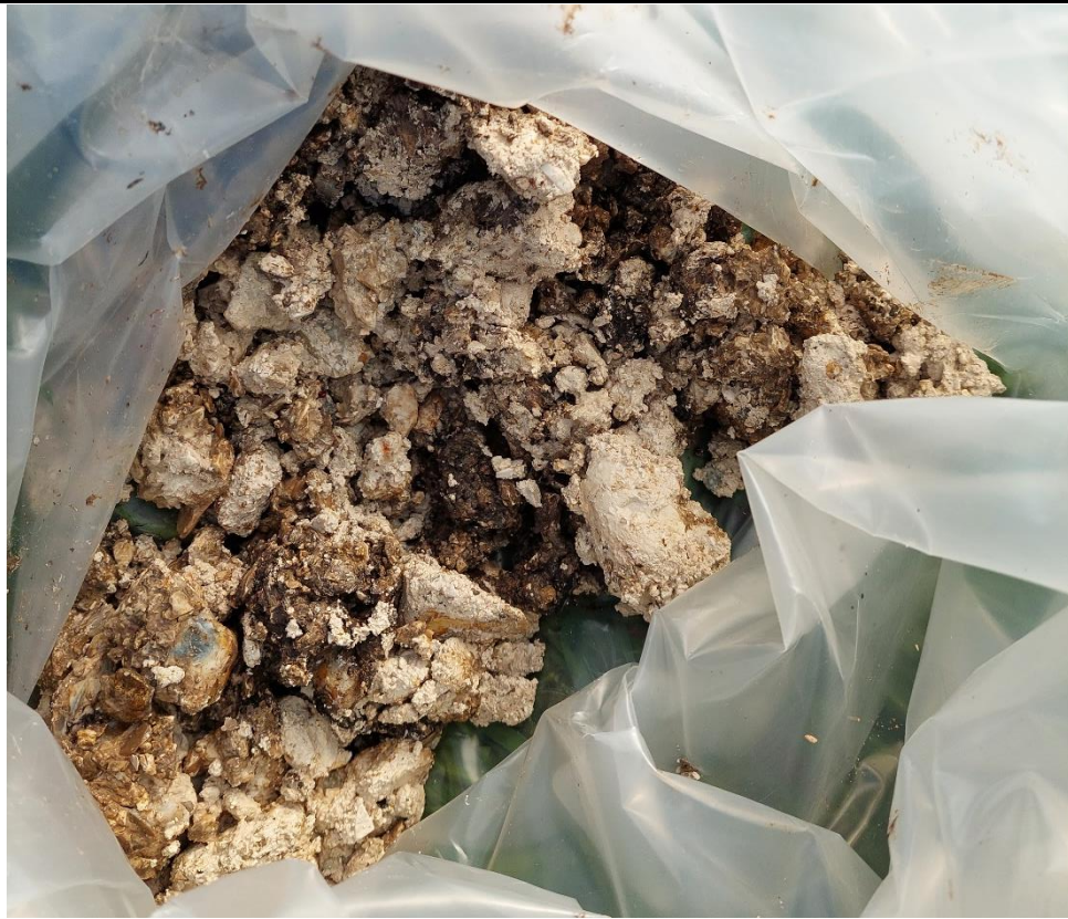
Chalk encountered at 1-1.2m bgl in BH04
