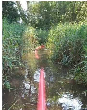
Temporary pipework in channel downstream of Riverside Cottages (12/08/2022)
