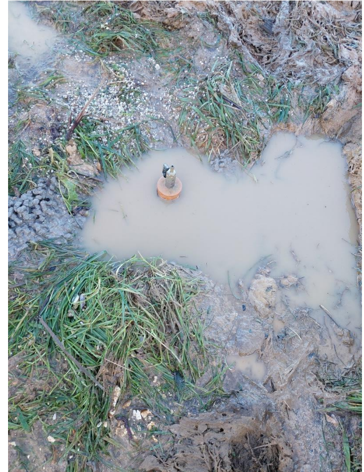
BHB01 prior to installation of headworks
