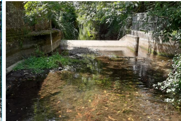
View downstream at Site 7, 21 l/s (31/08/2022)
