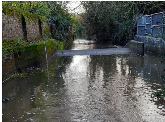
View downstream at Site 7, 122 l/s (08/11/2022)
