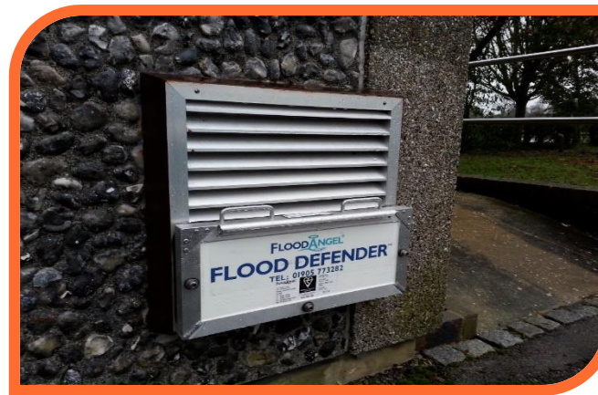
Figure 16 – flood protection of air vents at one of our sites
