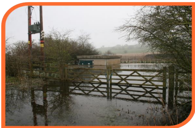
Figure 15 - flooding at a pumping station
