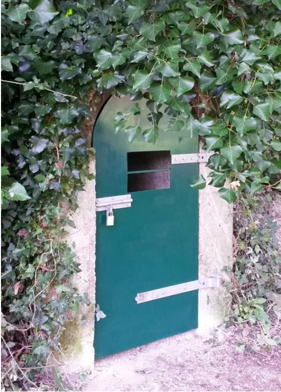
Photo 3: Bat roost created at Northbrook WTW
