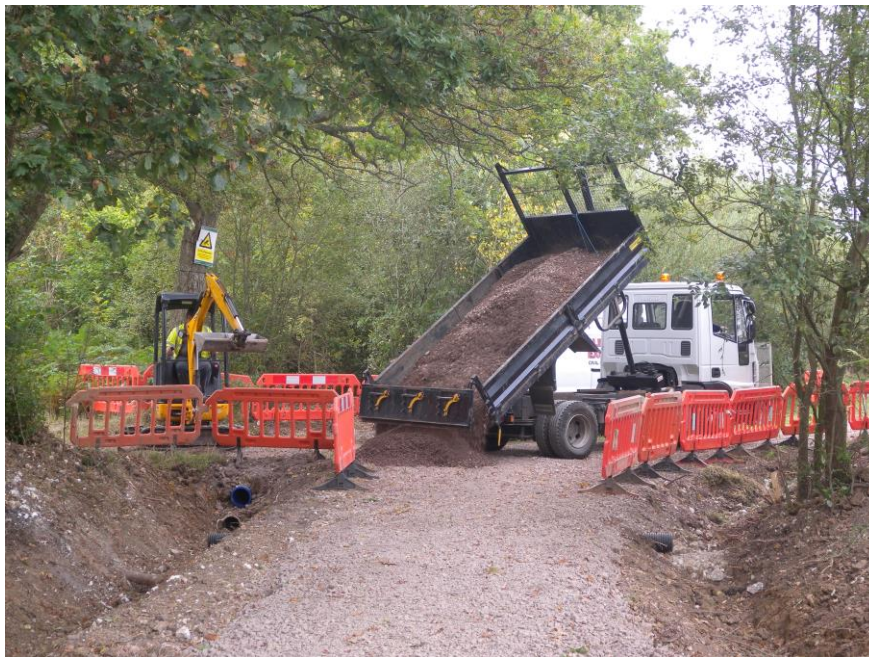
West path improvement works at Havant Thicket (September 2014)
