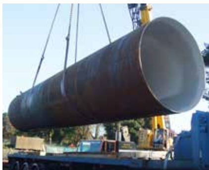
Relining of the well at Eastergate Pumping Station
