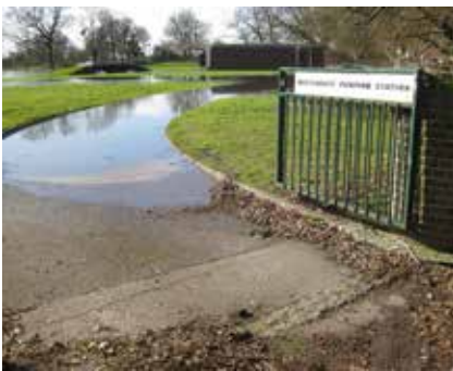
Flooding at Westergate Pumping Station caused by one of the wettest winters on record in 2014
