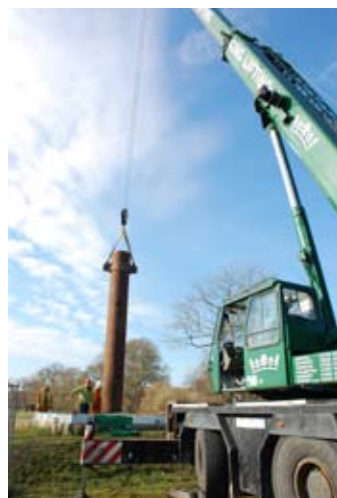
RIGHT Borehole relining at Walderton Water Treatment Works
