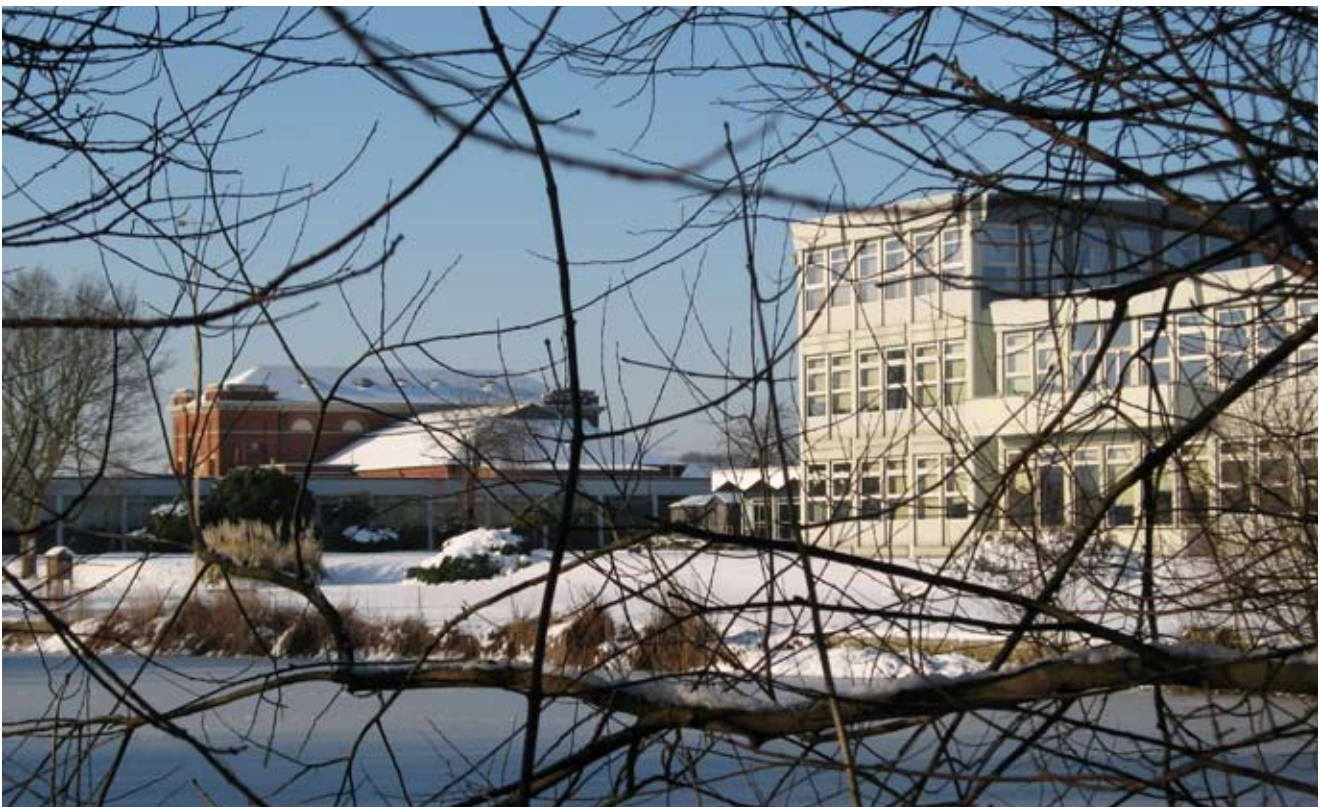
Havant Head Office and Pumping Station taken in the snow in January 2010
