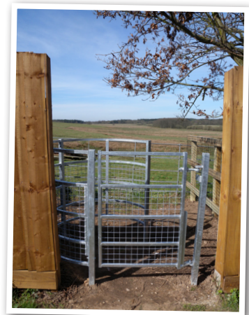
New kissing gate & boundary fence
