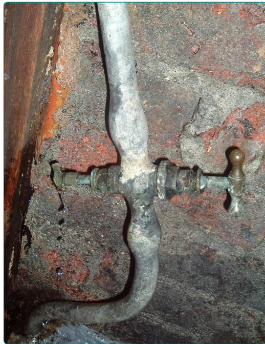
Figure 5 – Example lead pipe arrangement
