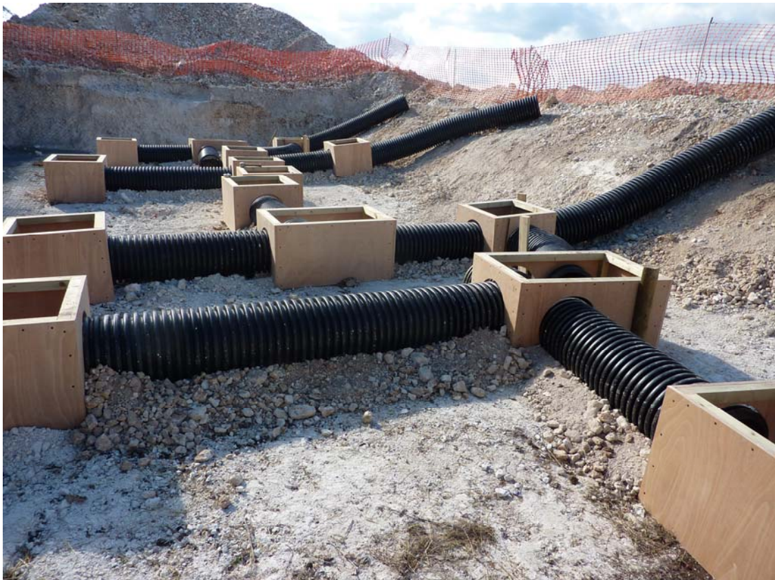
Construction of an artificial badger sett on Portsdown Hill
