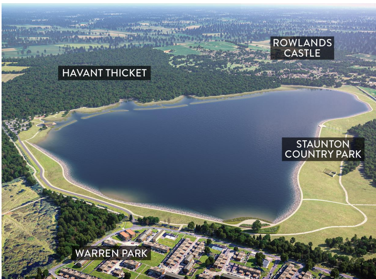
Figure 1: The Havant Thicket Reservoir
