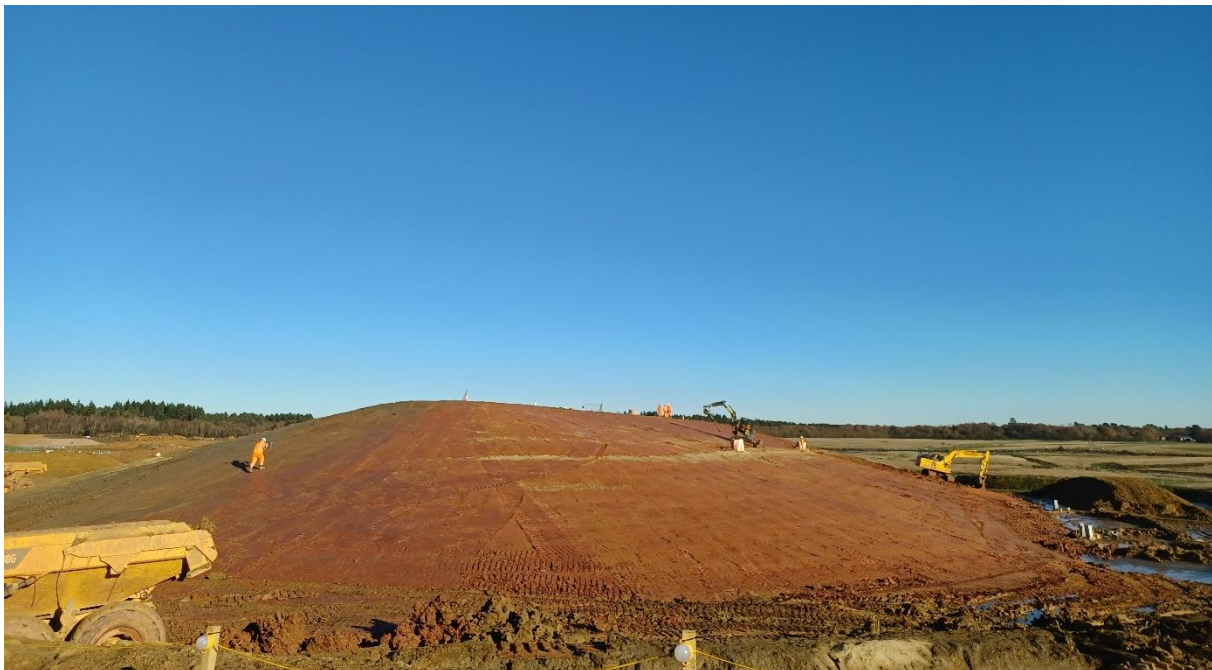
Figure 5: Trial embankment at the Havant Thicket Reservoir construction site
