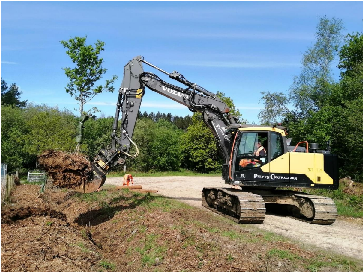
Figure 2: Tree translocation at the Havant Thicket Reservoir construction site
